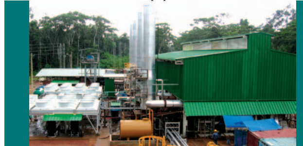
Pluspetrol & Ferrenergy, 4 x 16PA6B gen sets de combustible pesado, Peru
