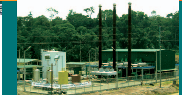
Dygoil 3 x Cat® 6CM25 engines, 5.2MW Ecuador
